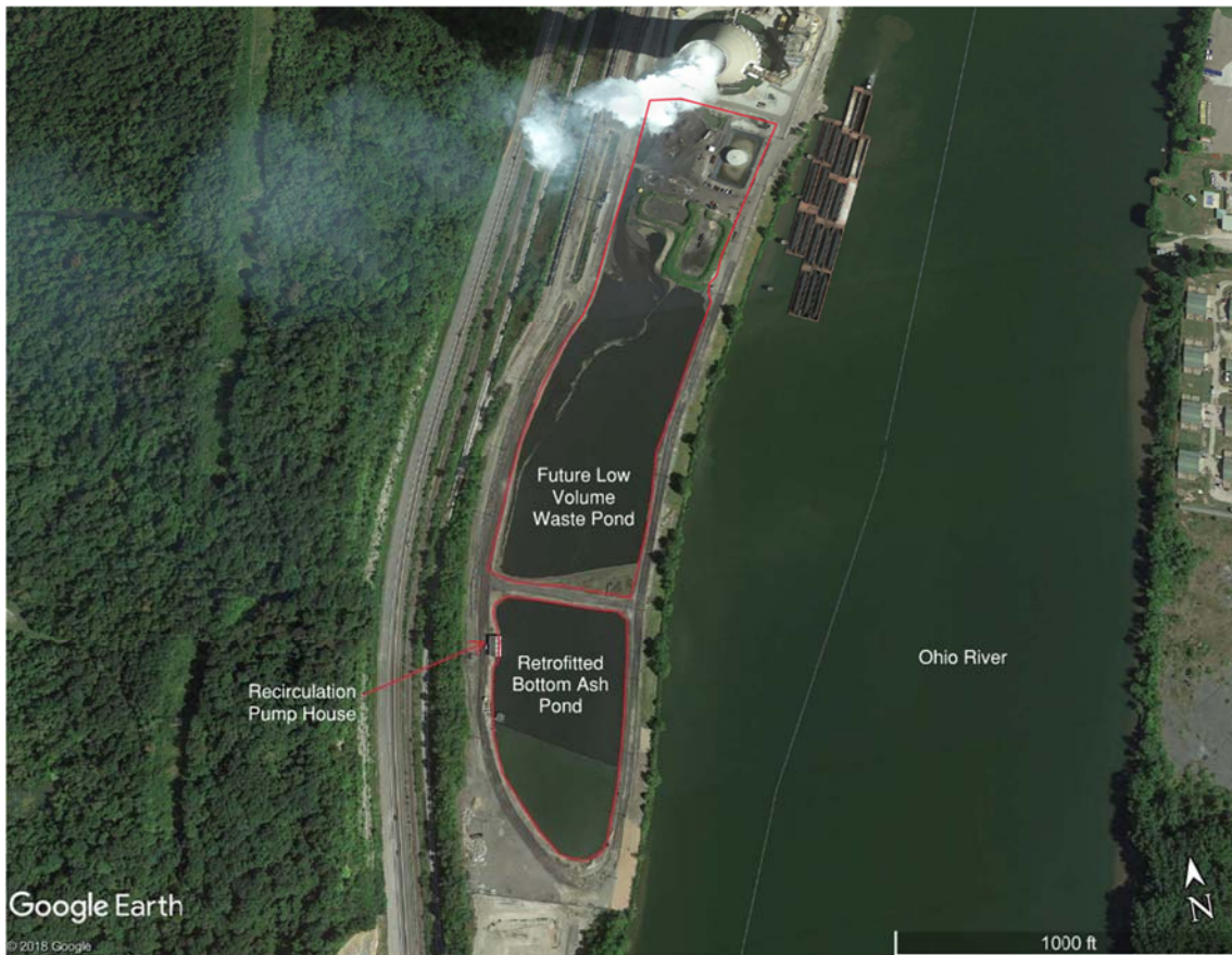
Figure 1 – Aerial View of the Cardinal Power Plant Bottom Ash Complex
